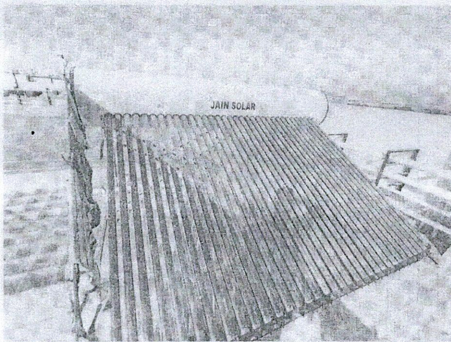
Solar Water Heater
