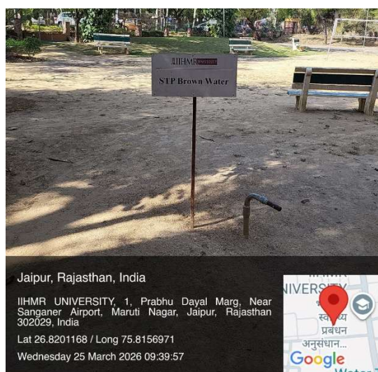
STP Treated Water Reuse for Landscape Irrigation
