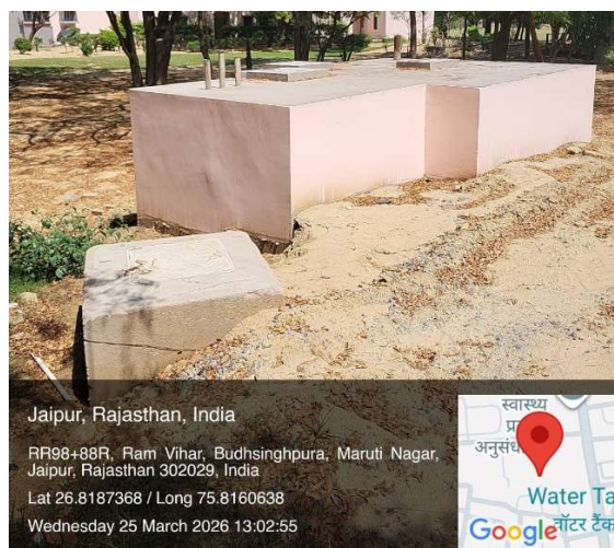
Rainwater Harvesting Recharge Structure
