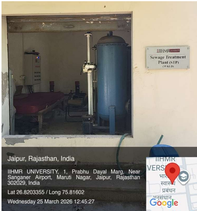
35 KLD Sewage Treatment Plant (Operational)
