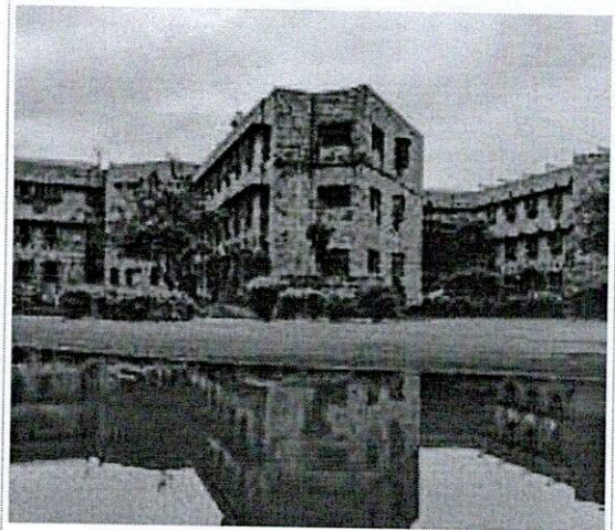
Pond for rainwater recharge
