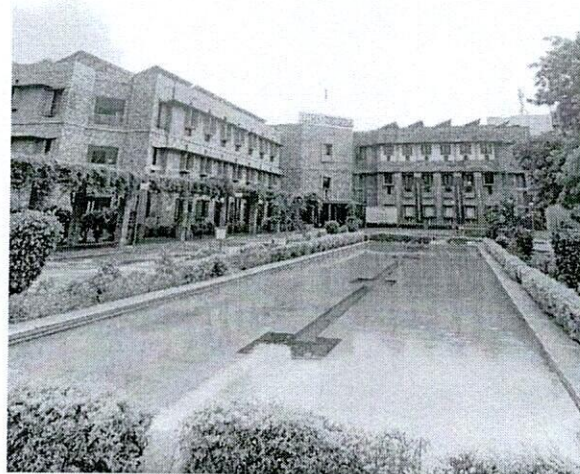
Rainwater Harvesting Artificial Pond
