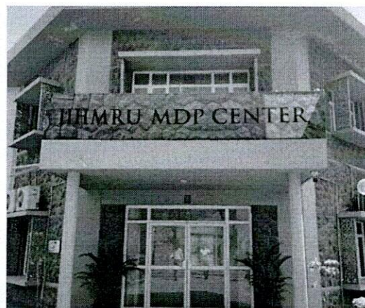
Well Ventilated Building
